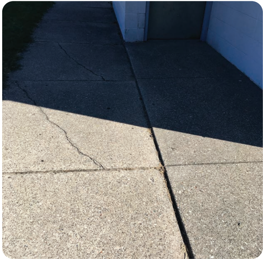
Pavement around restroom building is cracked and settling. Restroom building is in good condition.
