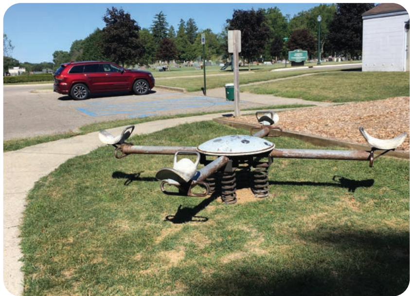
Play equipment is missing required safety surfacing.
