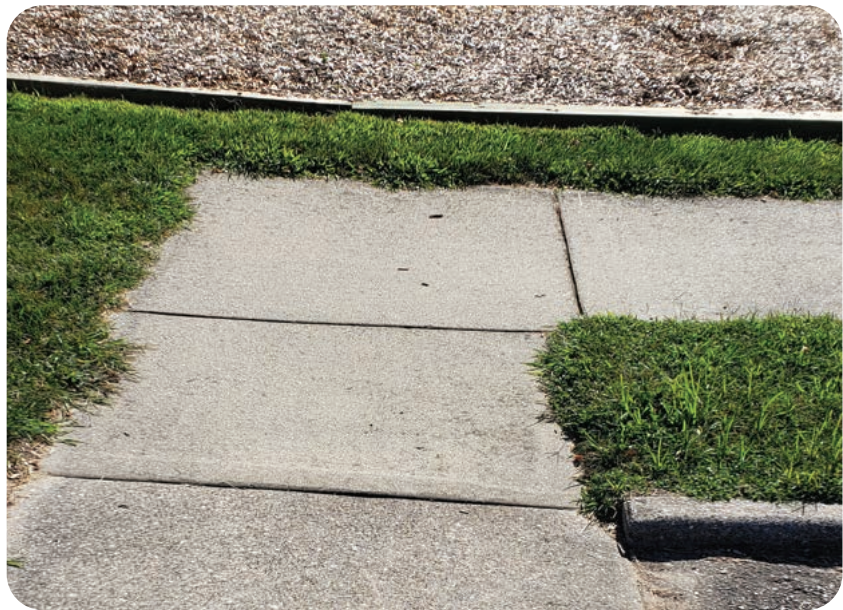
Portion of walkway exceeds maximum slope for barrier free accessibility.
