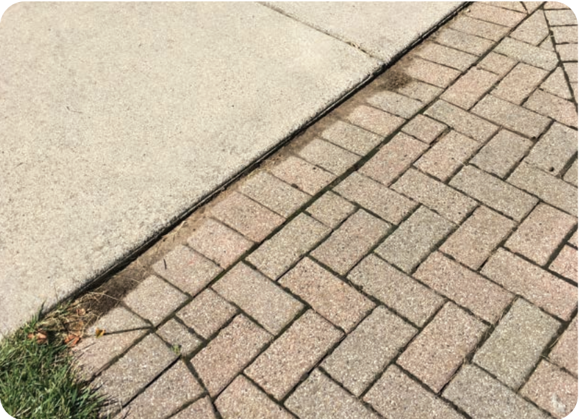
Pavers are aesthetically pleasing, however, trip hazards at transition areas need to be replaced.
