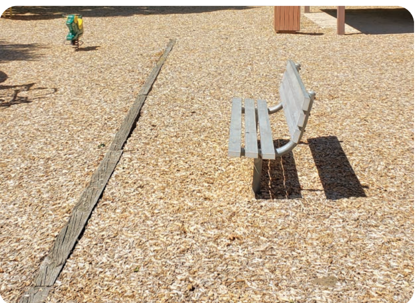
Bench lacks barrier free route. Also none of the benches have companion spaces.
