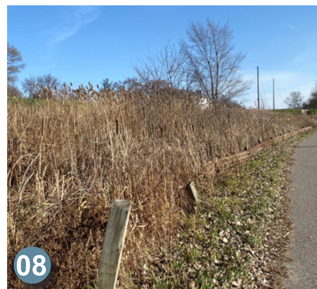
08 Shoulder of road is steep and swale has wetland like plantings.
