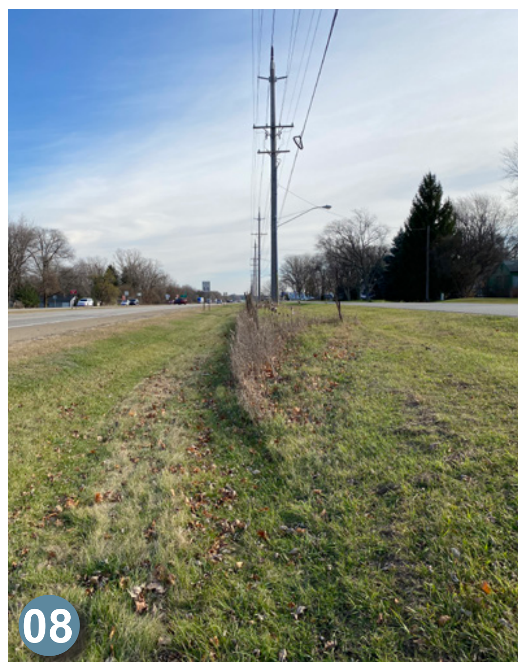
08 View east showing utility poles and wire fencing.
