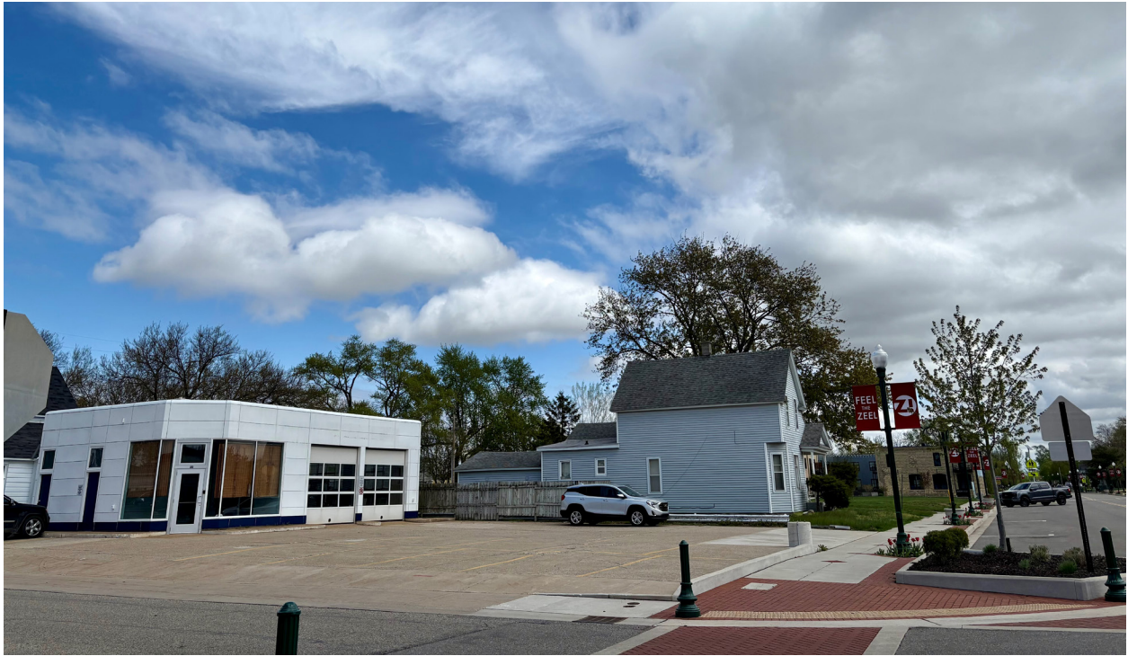
303 E. Main property looking east along the north side of E. Main Avenue.
