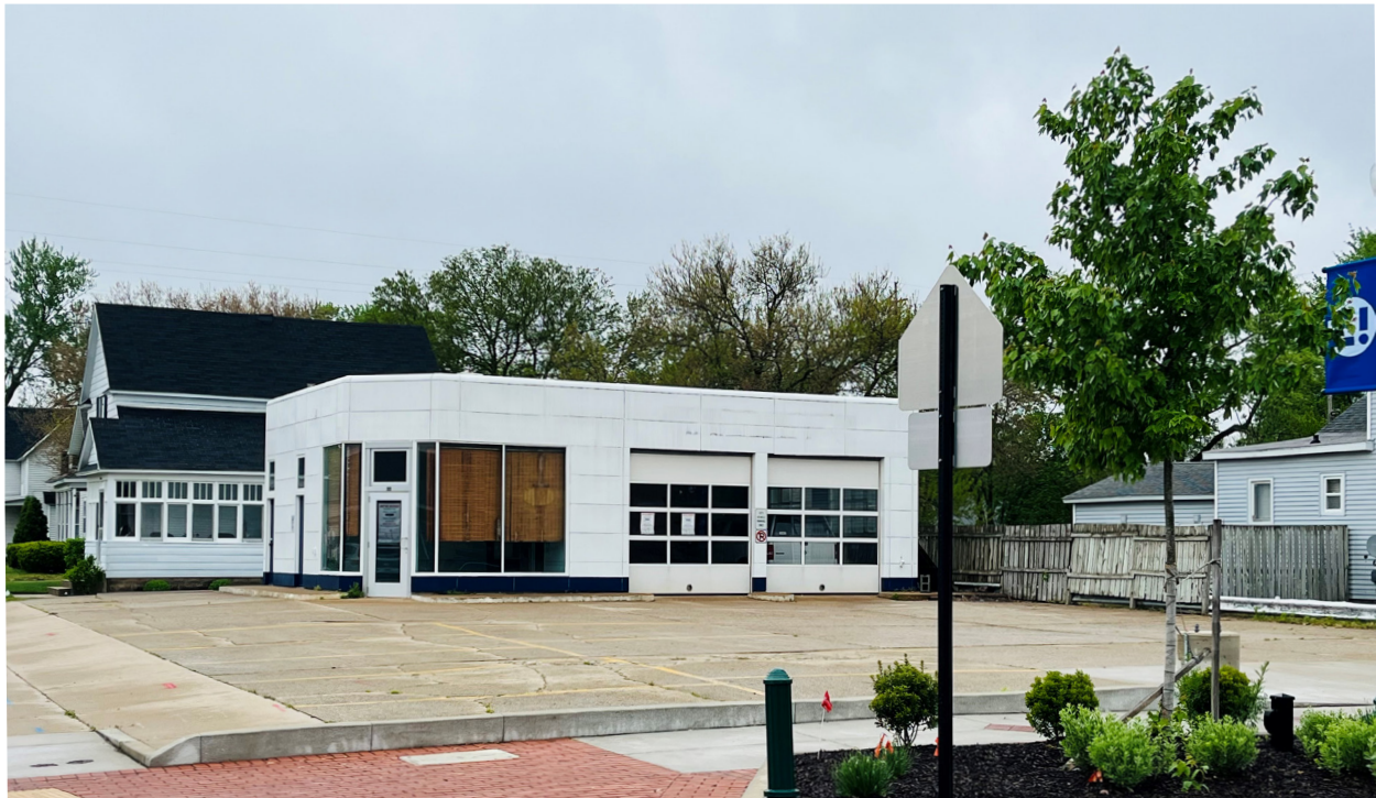
303 E. Main property from E. Main Avenue.
