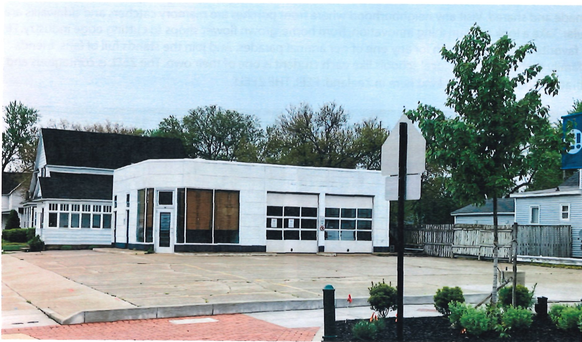
303 E. Main property from E. Main Avenue.
