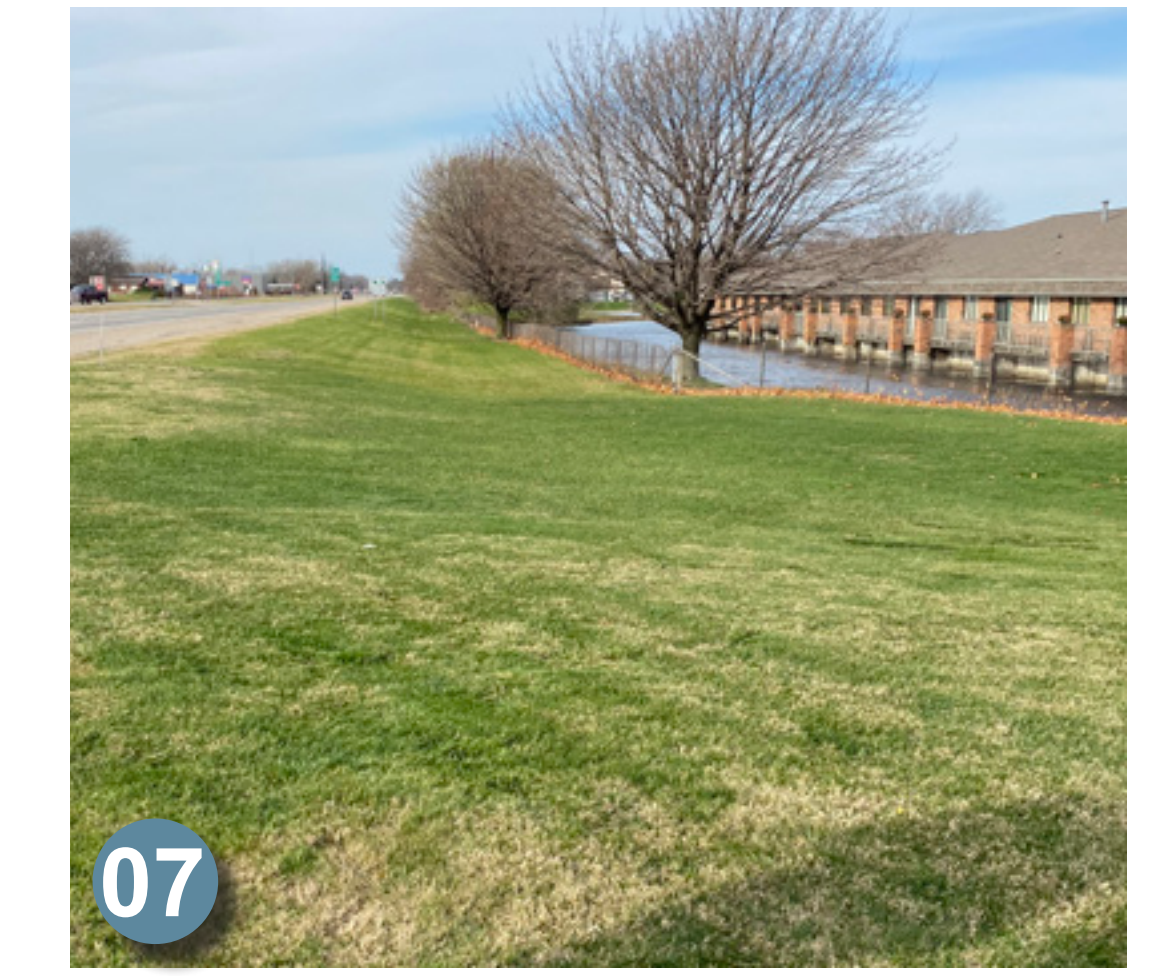
07 View to pond is attractive, however, fencing collects unsightly debris.
