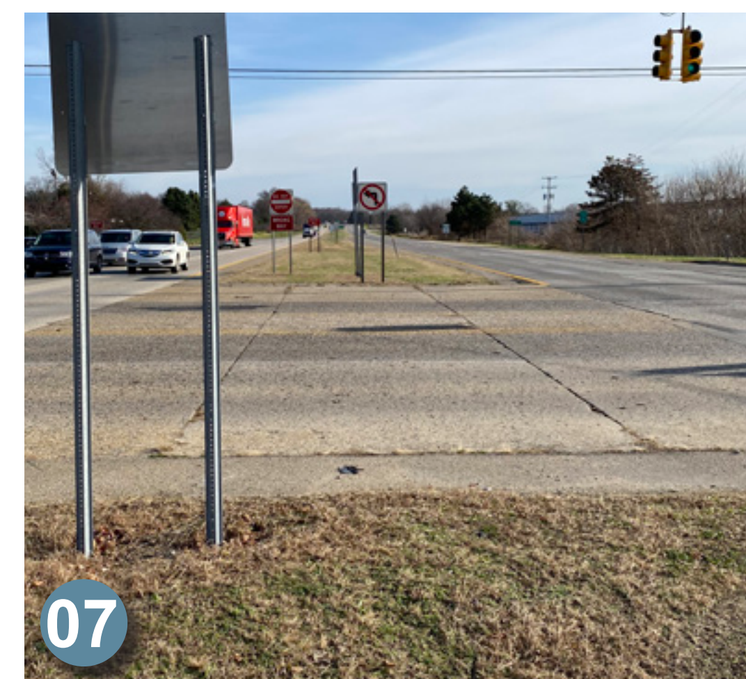
07 View looking East down median. This portion of the median is relatively flat and open, except for signage. However, due to federal and MDOT standards, improvements are limited to low growing plant material and breakaway items.
