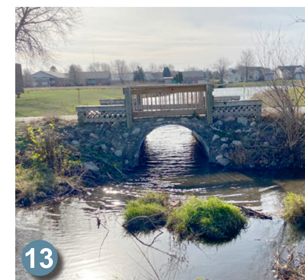
13 Culvert/bridge crossing at adjacent, non-motorized trail.
