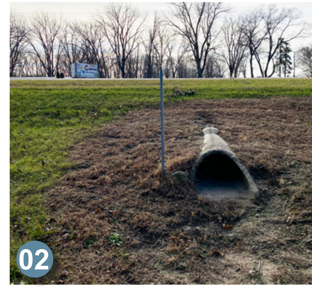
02 Culvert under road for storm water drainage.
