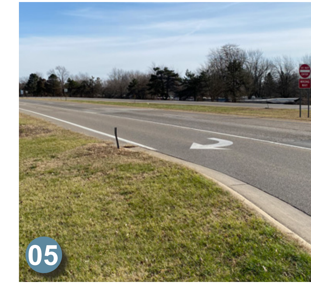
05 View looking East. Shows open and flat median with steep shoulders on North and South side of the road.
