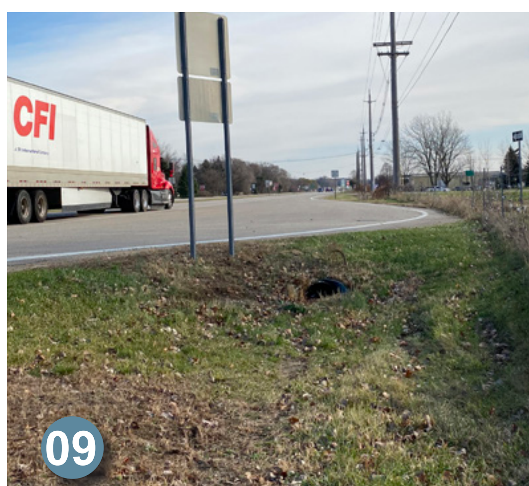
09 Typical bump-out for turning trucks. Culvert shown here to allow for storm water drainage.
