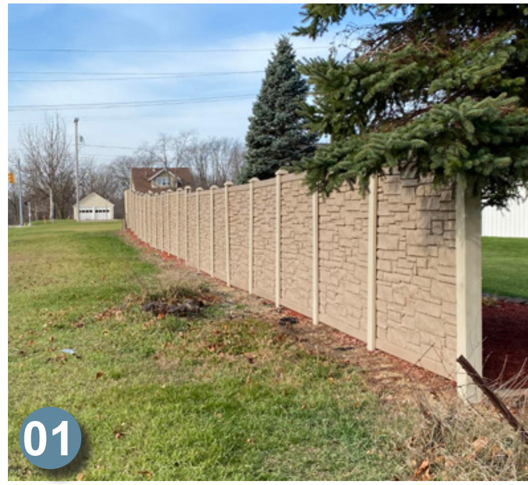
01 Privacy fencing along right of way to block views to residents. Open lawn area is in clear vision triangle for intersection.
