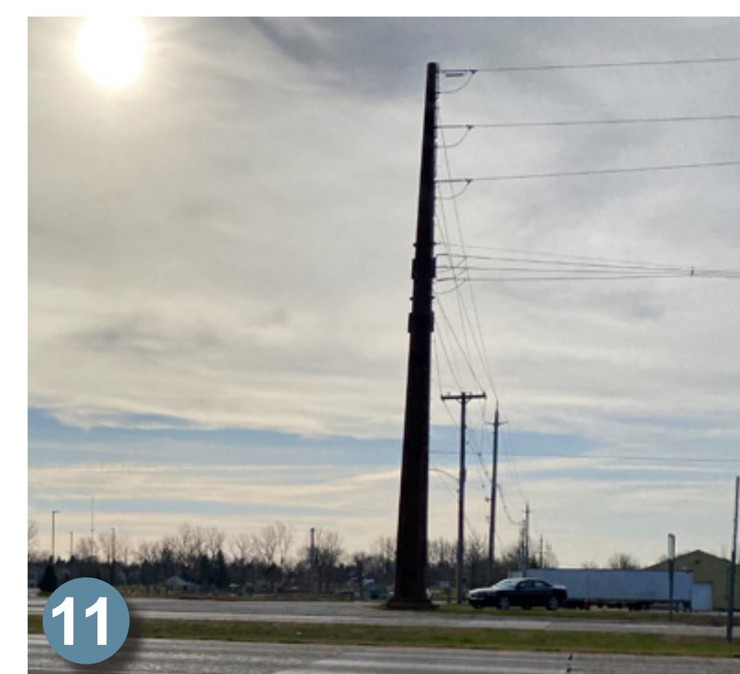
11 Large utility poles along the right of way.
