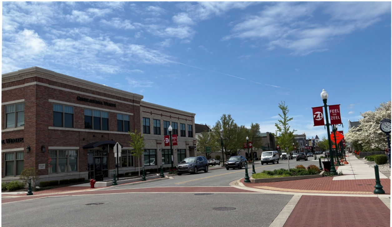
303 E. Main property looking west along the south side of E. Main Avenue.
