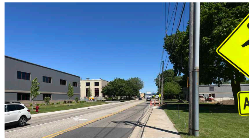
Overhead utilities on the south side of E. Washington Avenue.
