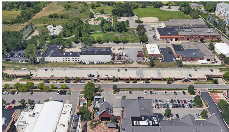
A linear single-level parking deck situated along 7th Street in Holland, Michigan provides additional parking for the downtown area.
