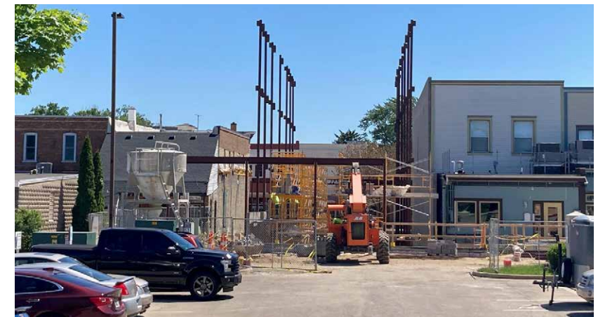
135/137 E. Main Avenue development and passageway project
