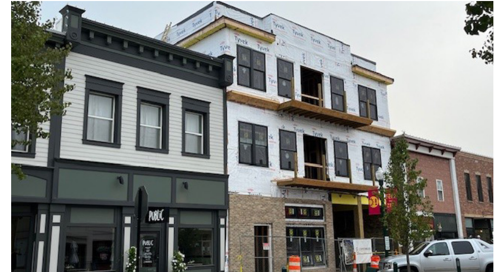
Progress on the 135-137 E. Main Avenue project.
