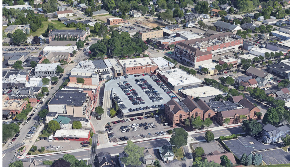
A single-level parking deck situated behind Main Street supports Plymouth, Michigan’s vibrant downtown area.
